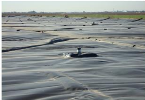
Covered Lagoon Digester
