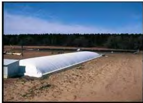
Plug-Flow Digester
