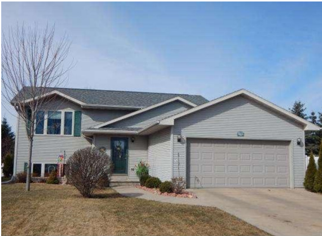
RESIDENCE - Bi-Level_ Grade C
