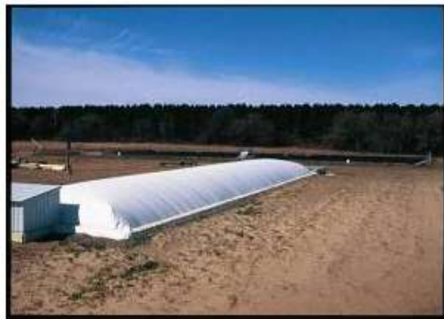
Plug-Flow Digester
