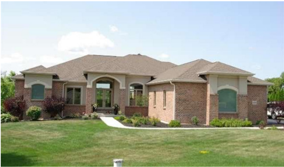
RESIDENCE - Modern Single Story_ Grade B plus (+)
