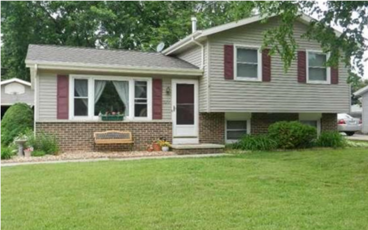
RESIDENCE - Split-Level_ Grade C minus (-)
