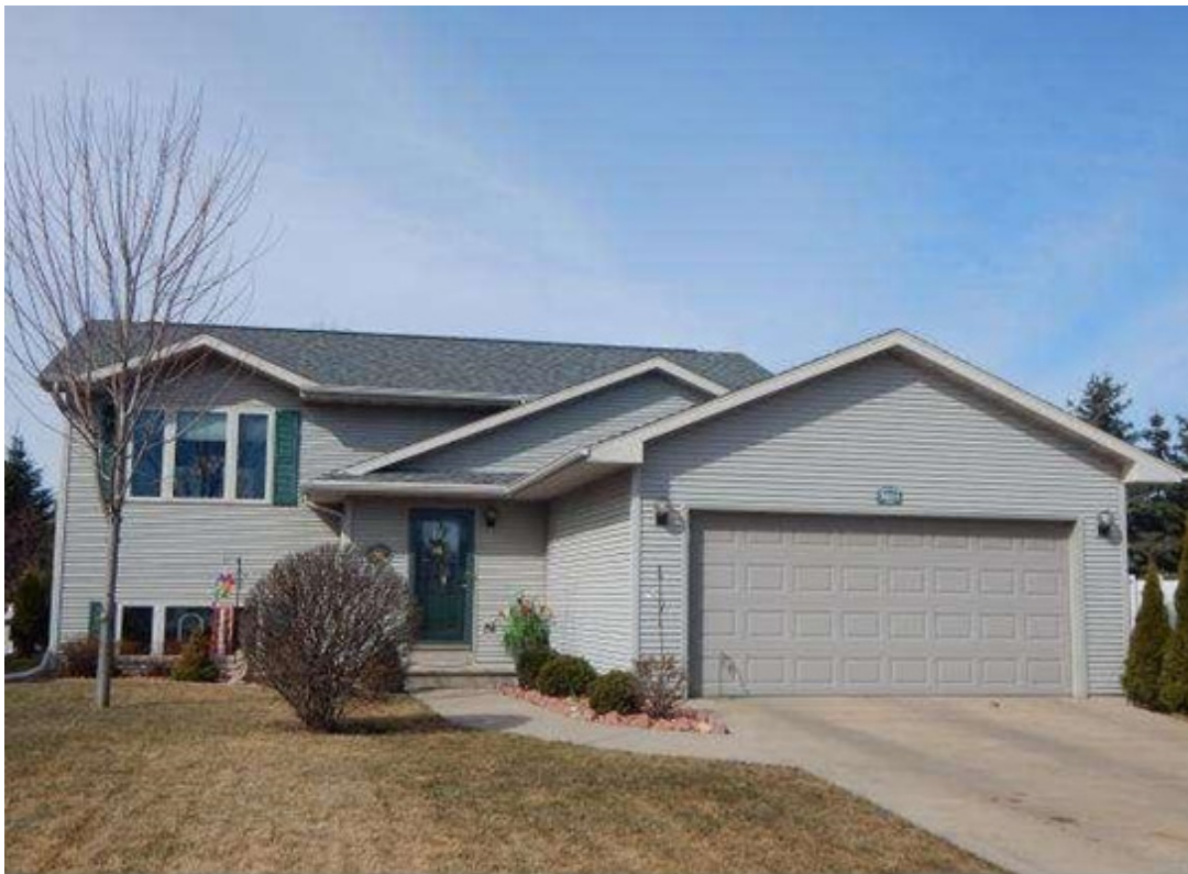
RESIDENCE - Bi-Level_ Grade C
