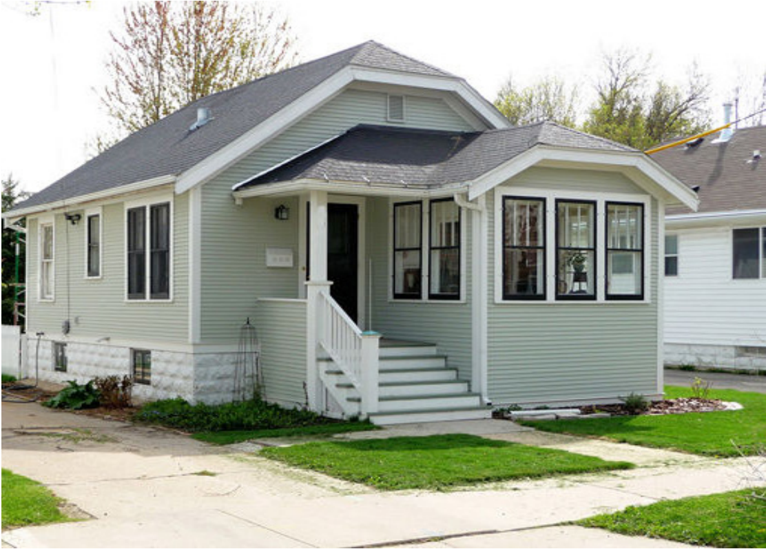
RESIDENCE - Bungalow_ Grade D
