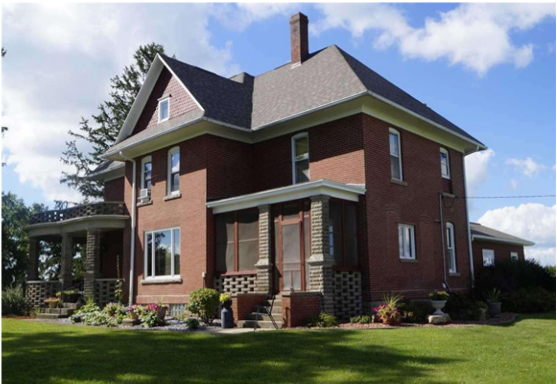
RESIDENCE - Farmhouse_ Grade B
