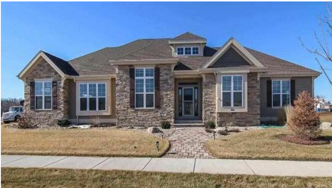
RESIDENCE - Modern Single Story _Grade B plus (+)
