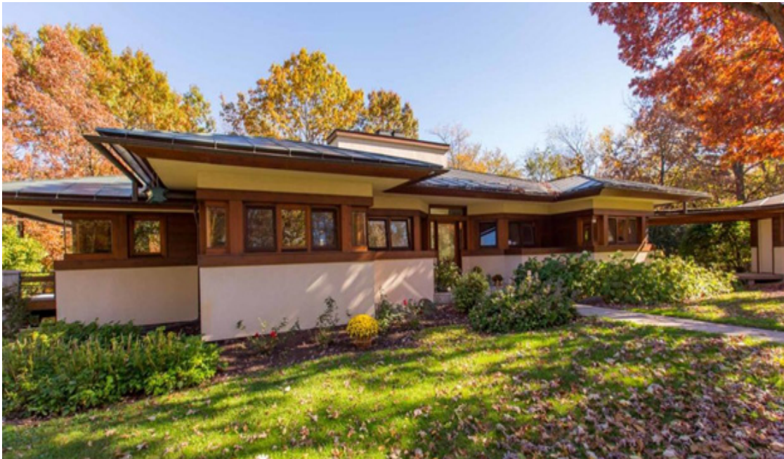
RESIDENCE - Prairie_ Grade A
