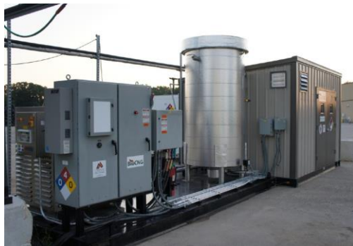
BIO CNG System CNG Pumps
