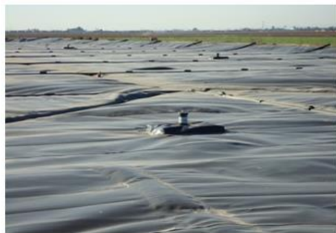
Covered Lagoon Digester
