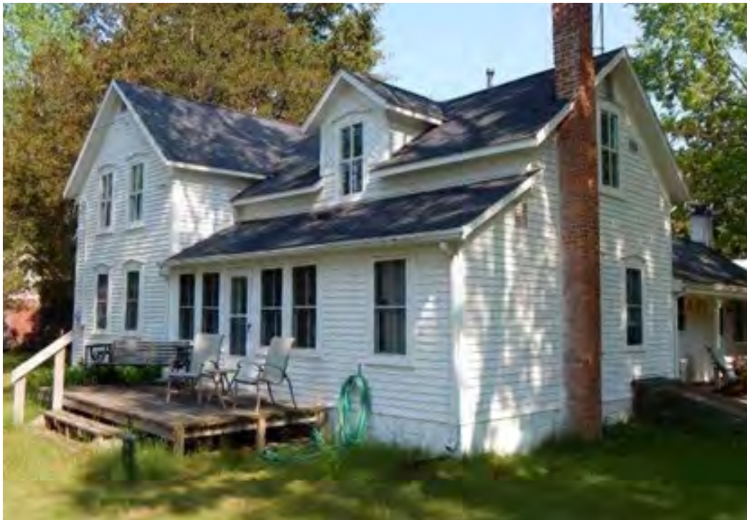
RESIDENCE - Farmhouse_ Grade D
