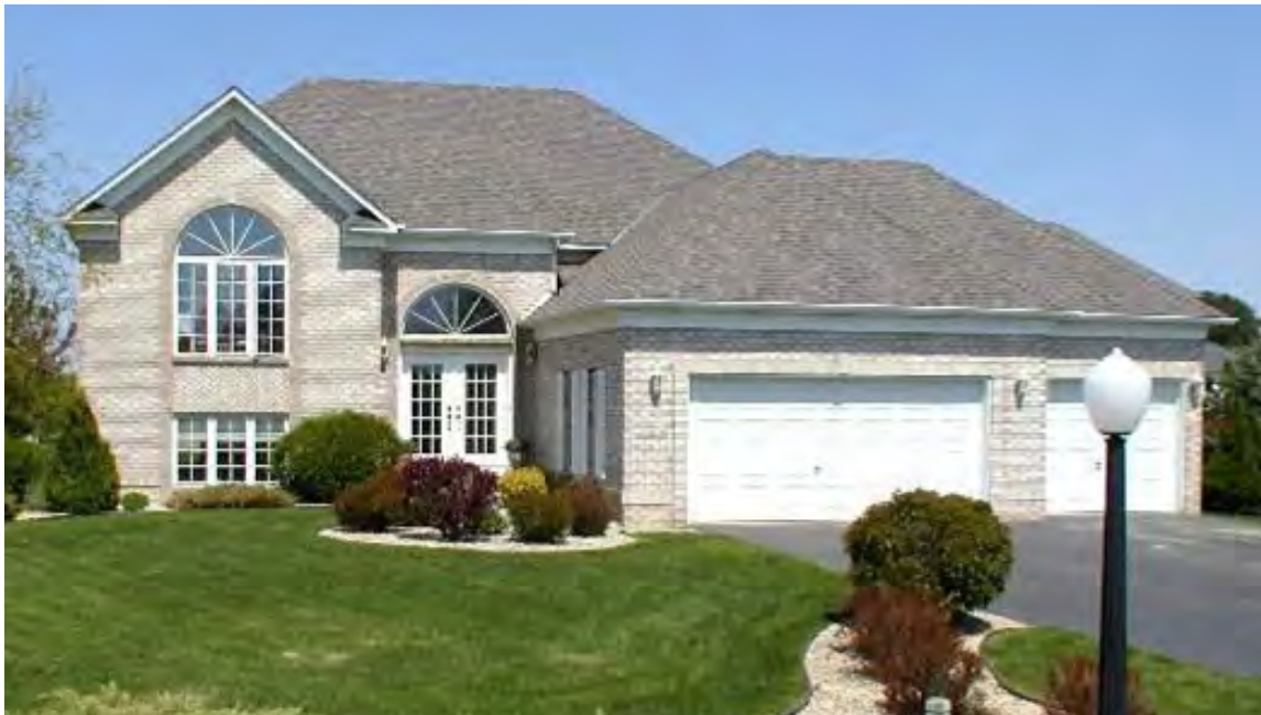
RESIDENCE - Split-Level_ Grade B plus (+)
