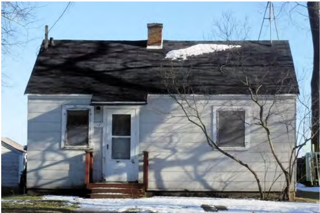
RESIDENCE - Cottage_ Grade E
