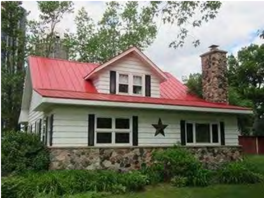
RESIDENCE - Farmhouse_ Grade D plus (+)
