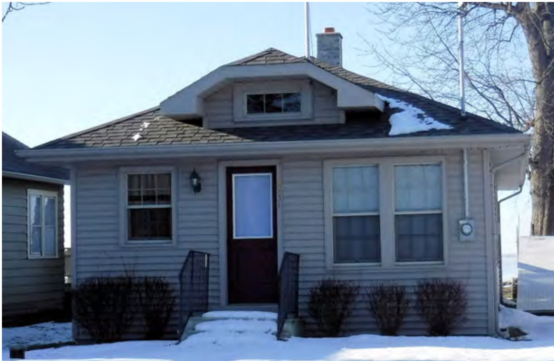
RESIDENCE - Cottage_ Grade D plus (+)
