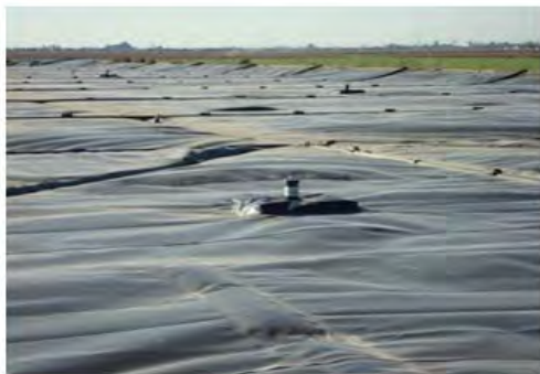
Covered Lagoon Digester
