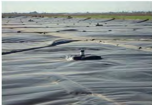
Covered Lagoon Digester
